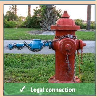
Approved hydrant backflow assembly in place.
